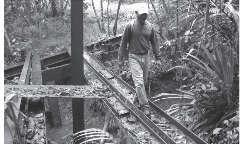
Above: Seacology is assisting the Palau Conservation Society (PCS) by funding the replacement of this old, slippery i-beam bridge in Palau's Ngaremlengui Nature Reserve with a covered bridge. Seacology is also funding three smaller foot bridges, as well as a welcome center for the reserve (photo credit: PCS).
