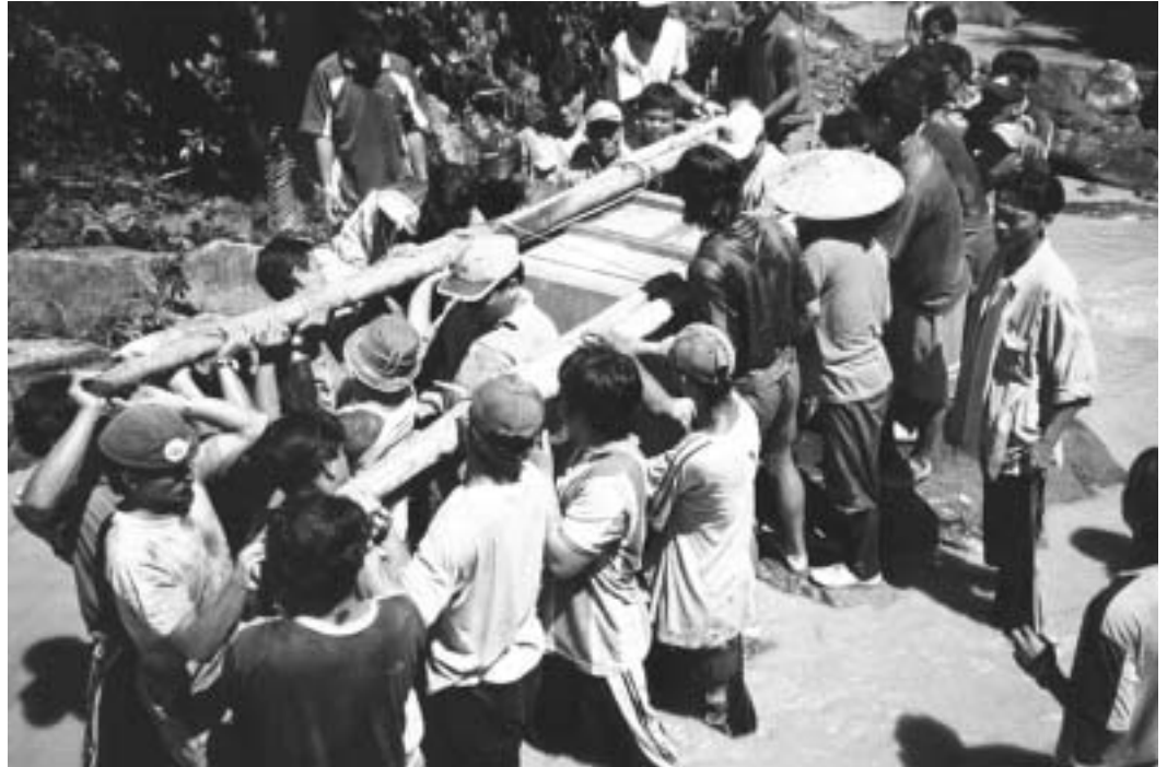
Working together, villagers from Long Lawen haul the turbo generator across the Selau River to the powerhouse.
